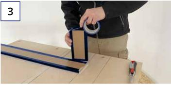
MASK THE DECOUPLING STRIPS Mask the cut edge only with Wolf tape. Allow the PhoneStrip tape to protrude by at least 2 cm at the corners.
