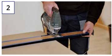
CUT THE DECOUPLING STRIP TO SIZE Hand-held circular saw with Widia blade & extraction Jigsaw with wood or metal saw blade, Cutter
