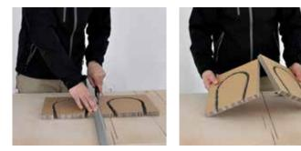
**RETURN LOOP AND EDGE FINISHING ELEMENTS** PowerFloor Light, Nature and Slim return loop and edge finishing elements can also be cut with a cutter on the front side.
